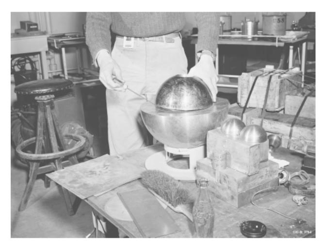
Figure 42. Configuration of beryllium reflector shells prior to the accident 21 May 1946.
