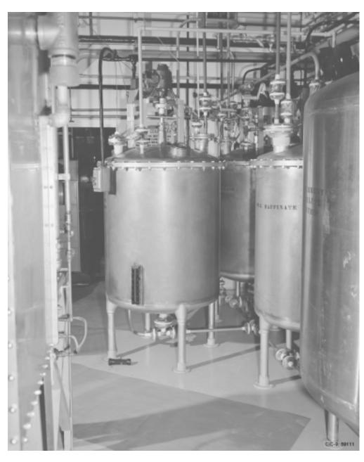
Figure 12. Vessel in which the 1958 Los Alamos process criticality accident occurred.
