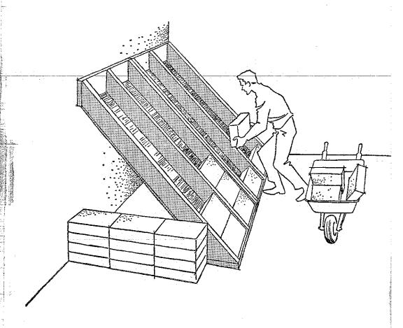
A simple and effective lean-to shelter can be built by constructing the components and storing them in your basement where they can be quickly assembled in an emergency. Components consist of a frame and filler materials, such as brick or blocks.
