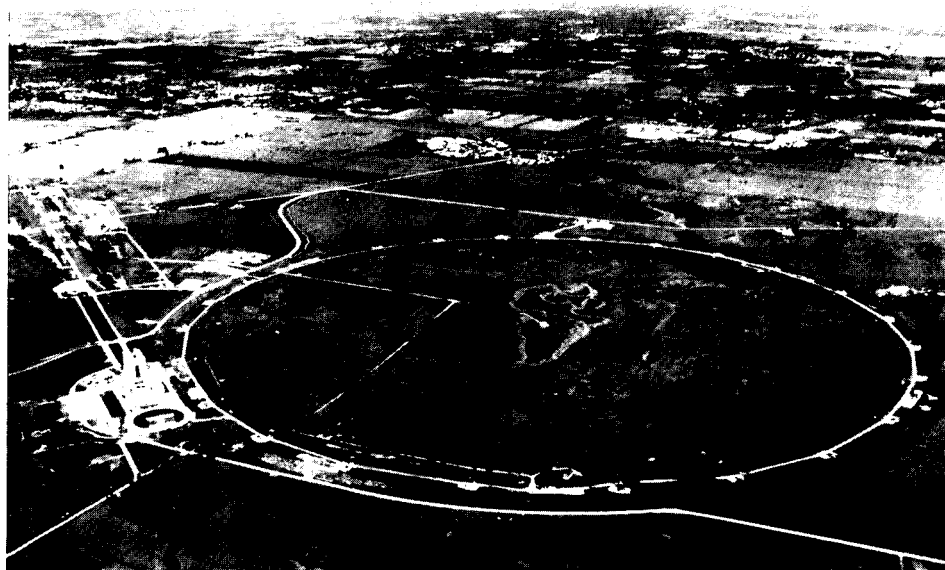
A state-of-the art version of a proton synchrotron. Here at Fermilab protons will be accelerated to an energy close to 1 TeV in a 6562-foot-diameter ring of superconducting magnets. Wilson Hall, headquarters of the laboratory and a fitting monument to a master accelerator builder, appears at the lower left. (Photo courtesy of Fermi National Accelerator Laboratory.)
